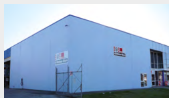
S&P-KRUGER AUSTRALIA S&P-KRUGER AUSTRALIA
