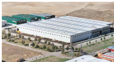
Planta Madrid Madrid Factory (Spain)
